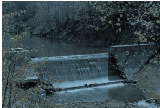
Figure 4.9(a): Concrete weir
