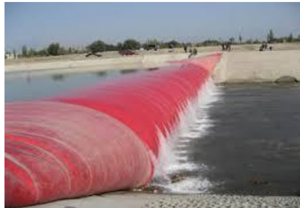
Figure 4.9(b): Inflated weir
